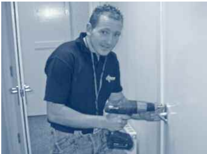
Working on repairs
